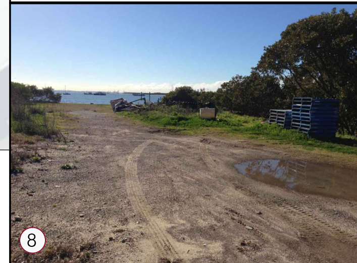
8 VIEW POINT - RECREATIONAL SPACE. WALL REBUILDING REQUIRED. BOARDWALK THROUGH MANGROVES.
