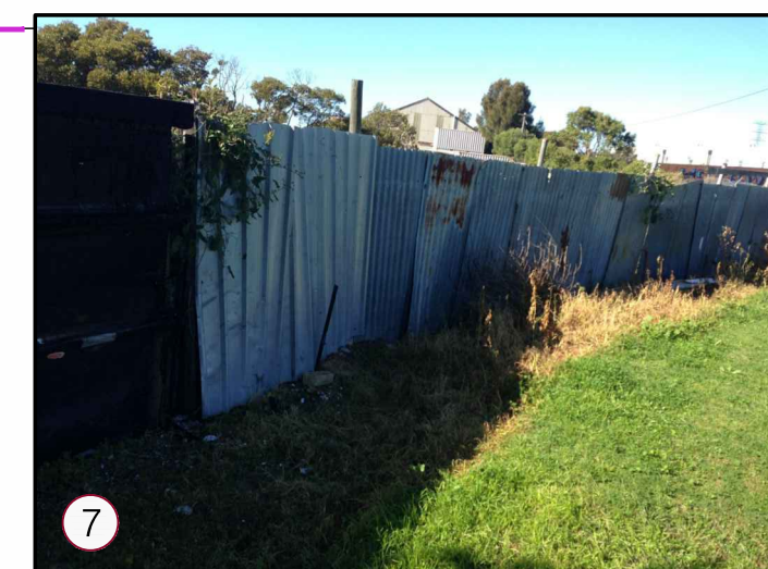
7 EXISTING FENCE ACTING AS A BARRIER BETWEEN TWO PROPERTIES.
