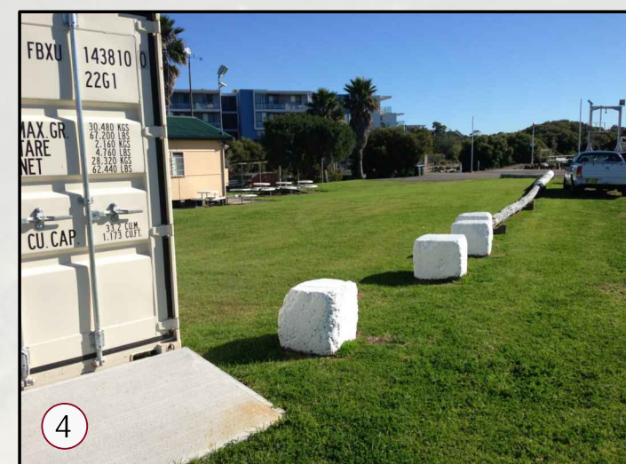
4 CONTINUE BOARDWALK ADJACENT TO STORAGE CONTAINER.
